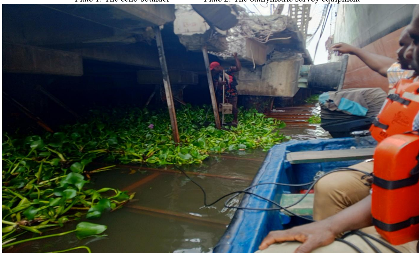
Plate 3. Echo sounding operation on-going / probing of the proposed pile point
